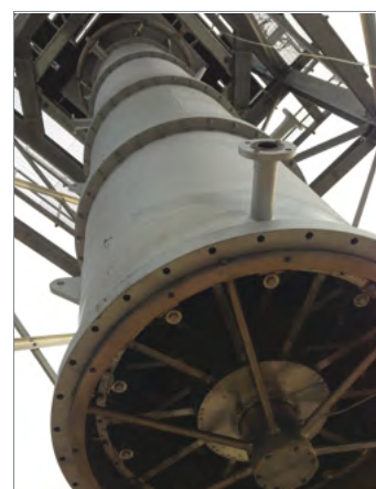
VERTICAL THIN FILM DRYER AS FINAL STEP OF ZLD PLANT
