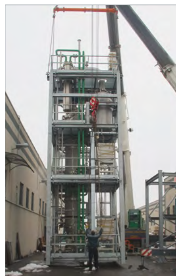
SINGLE EFFECT SKID-MOUNTED WIPED FILM DRYER FOR SALT DRYING
