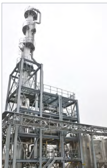
MULTIPURPOSE SOLVENT RECOVERY PLANT EQUIPPED WITH THIN FILM REBOILER
