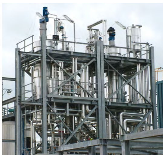
DOUBLE STAGE TFE-HHV SYSTEM FOR TDI REMOVAL FROM POLYURETHANE PRE-POLYMER
