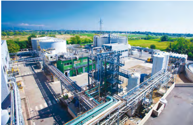
WASTEWATER & SLUDGE TREATMENT CENTER WITH SOLVENT RECOVERY SYSTEM & TOP WET OXIDATION REACTORS
